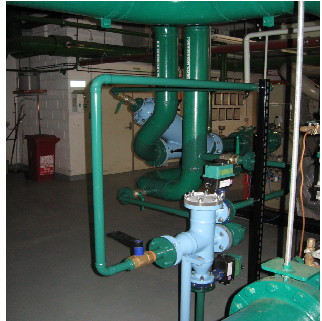
Fig. 3 The sponge ball ATCS installed in Case 1
